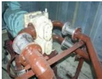
*Fig. 7 Provision of suitable dampers*
